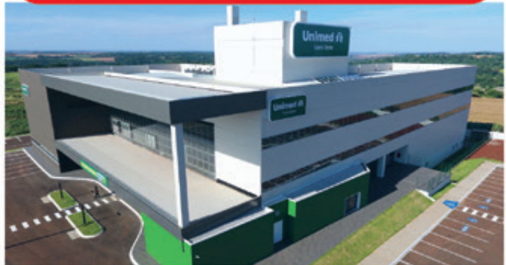
HOSPITAL UNIMED - MARECHAL CÂNDIDO RONDON-PR
